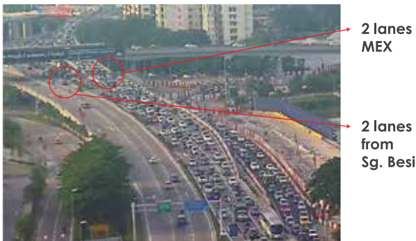
Figure 9: MEX Highway landing on Jalan Tun Razak. Lanes increased from 2 to 3 lanes for flow from MEX Highway / Jalan Sg. Besi on Jalan Tun Razak.
