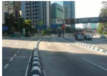
Figure 19: Physical barrier to overcome weaving problem near Double Tree Hilton.
