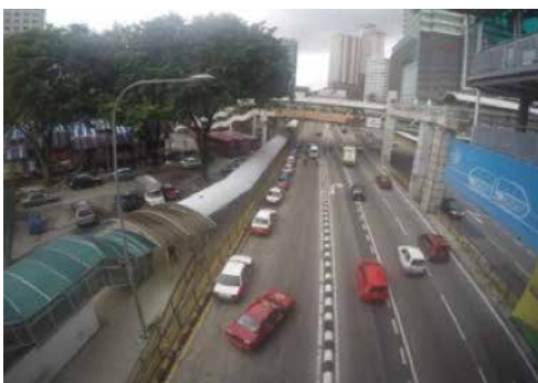
Figure 11: Physical barrier to overcome weaving problem near Titiwangsa Monorail Station
