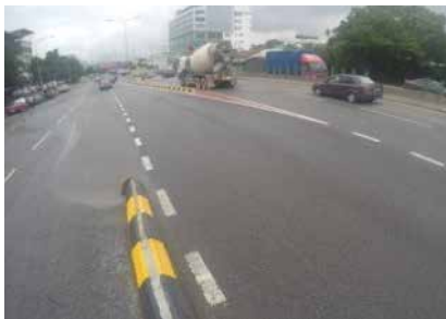
Figure 15: Physical barrier to overcome weaving problem in front of Fraser Park (Metro Pudu).
