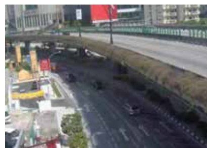
Figure 22: Reconfigure lanes on Jalan Tun Razak to accommodate an acceleration lane for AKLEH traffic.
