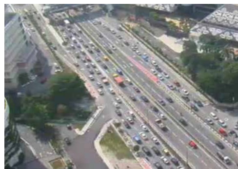
Figure 12: Physical barrier to overcome weaving problem in front of completed of IJN (North Bound).
